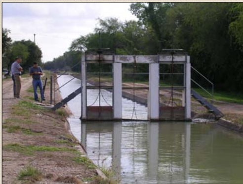
Figure 1. Bryan Canal Head Gates
