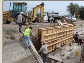
Constructing the new control structure
