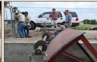
Installing and testing the new actuator
