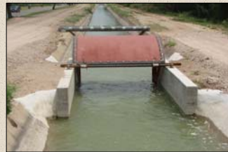
Installing the new gate
