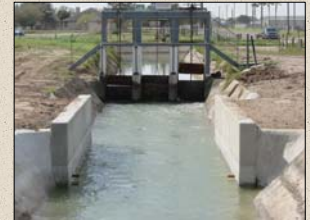
The new control structure is ready for the new radial gate
