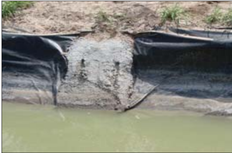
Figure 4. Concrete sections poured on top of a polypropylene liner
