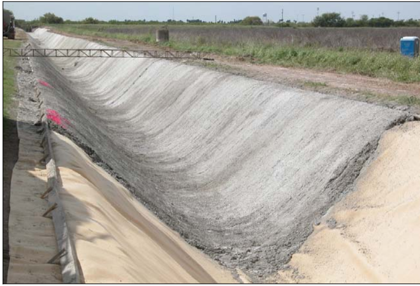
Figure 2. Polyester canal liner with a 3-inch protective barrier
