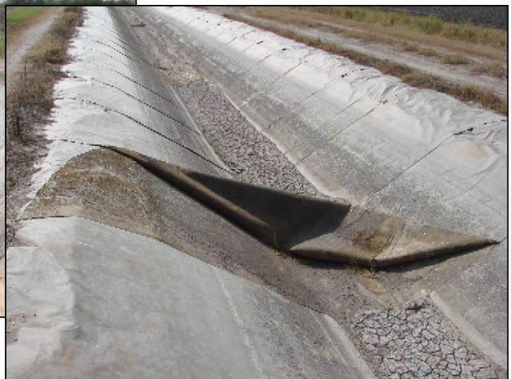
Liner has been torn and pulled off the canal sidewall
