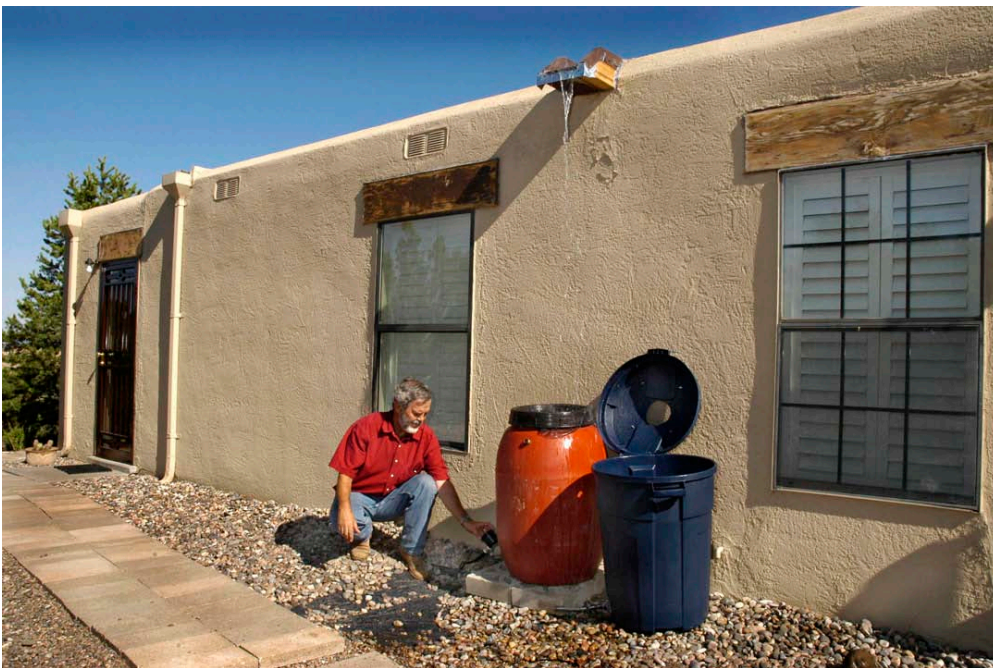
George Dickerson, horticulture specialist with NMSU's Cooperative Extension Service, demonstrates how roof water flows to rain barrels below to catch runoff for irrigation. The factory-made orange barrel cost Dickerson $60, but the black barrel is a trash bin he converted to a rain barrel for less than $20.
