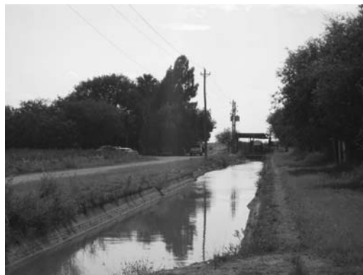
Figure 7. Ground-level photograph of a concrete canal section in the Delta Lake Irrigation District (Case 2)
